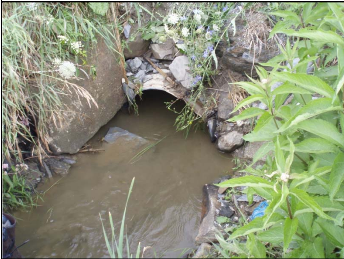
Photo 1. Upstream of culvert
