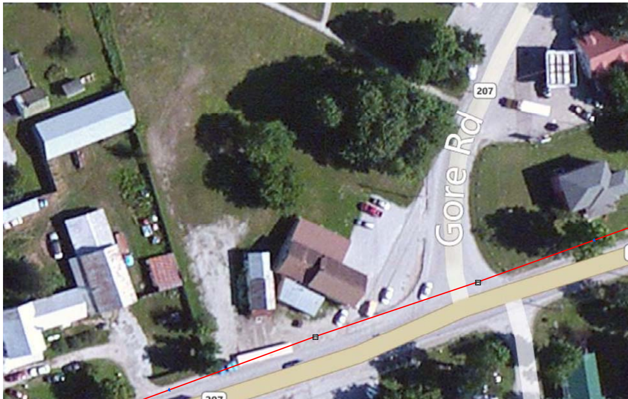
Figure 5. The Highgate Municipal Town Plan proposes the construction of a Park-and-Ride facility at the corner of Vermont Routes 207 and 78. Soil conditions favor infiltration-based practices, such as porous pavement, at this site.
