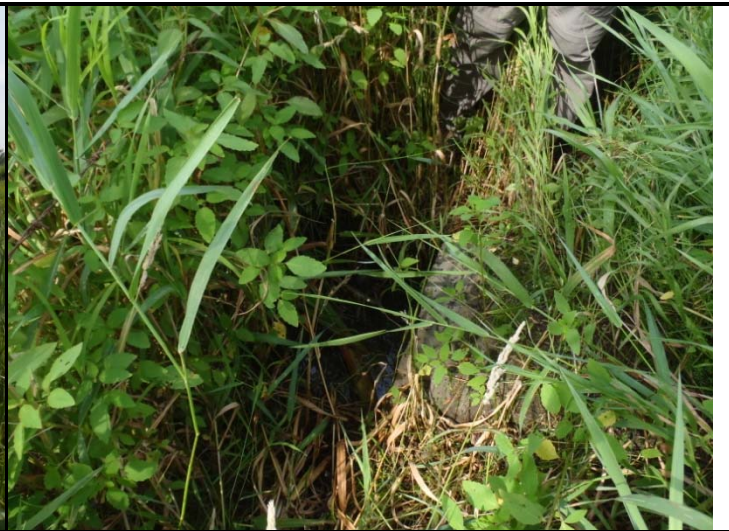
Photo 2. Downstream of culvert
