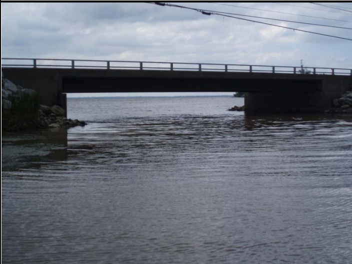
Photo 1. Route 7 bridge over the Rock River
