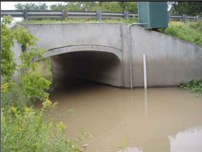
Photo 1. Downstream of bridge
