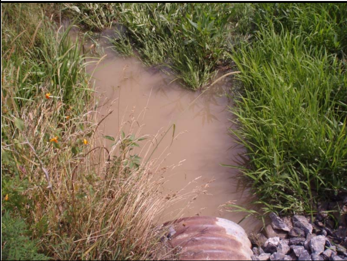
Photo 1. Upstream of farm road bridge
