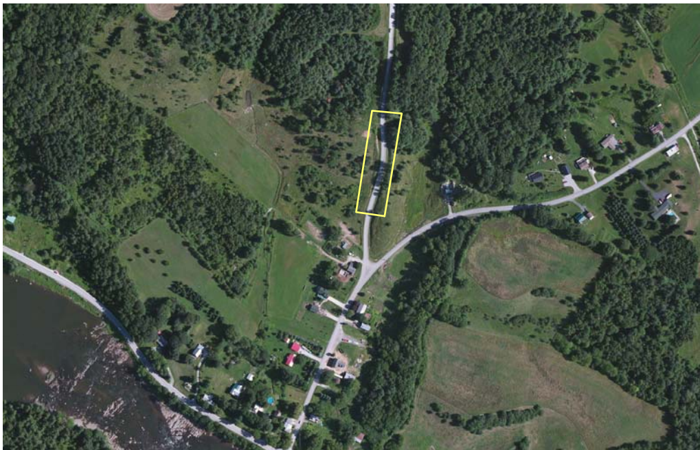
Figure 1. An area of eroding slopes along Durkee Road is highlighted in yellow.
