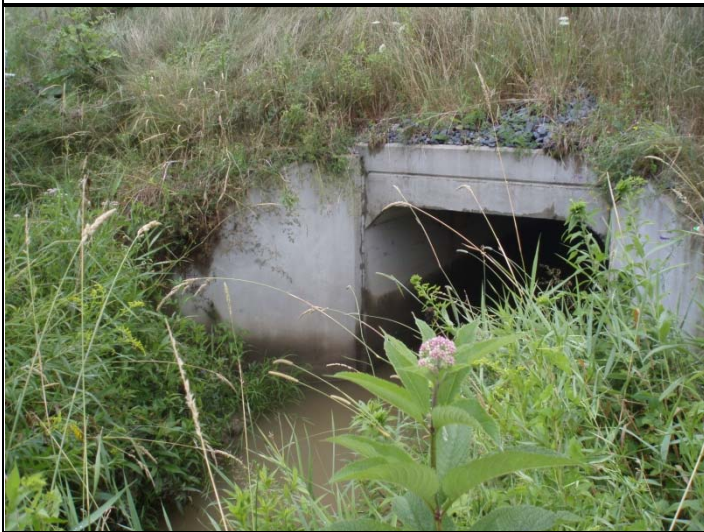
Photo 1. Downstream of bridge
