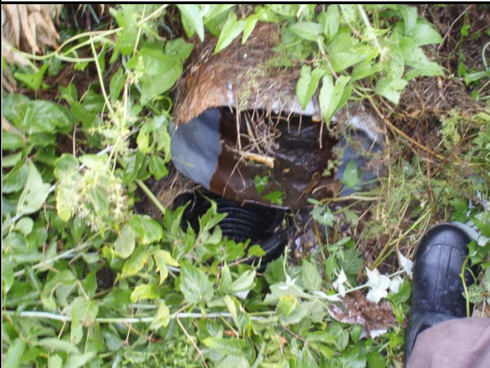
Photo 1. Downstream culvert drains to pipe
