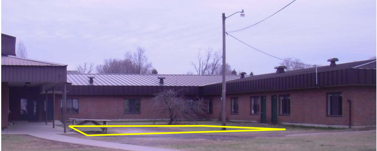
Figure 7. A large rain garden or bioretention area could be installed in the rear courtyard of the school where green space is not currently utilized.
