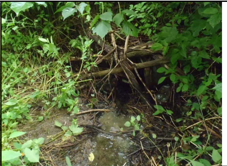
Photo 2. Outfall N of Brosseau Rd
