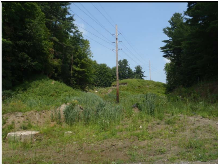
Photo 1. Landslide area from access road
