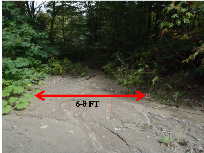
Figure 18. Eroding sediment from the road entering tributary to Missisquoi River.
