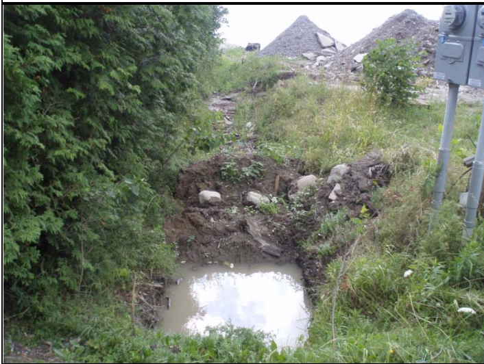
Photo 1. Potential culvert outfall area
