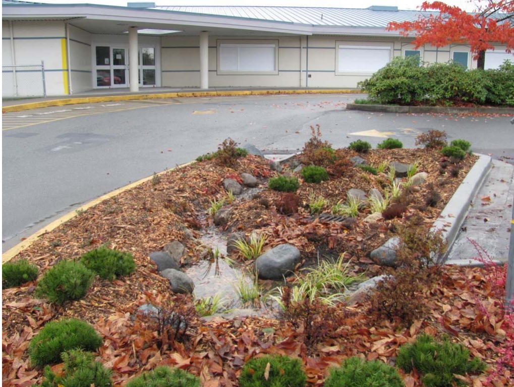
Figure 9. Example of a parking island being used to treat stormwater (Photo source: Cougar Creek Streamkeepers, http://www.vcn.bc.ca/cougarcr/raingardensrichardson.html ).
