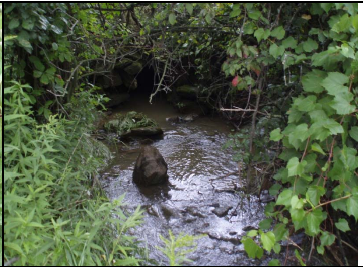
Photo 2. Downstream of culvert
