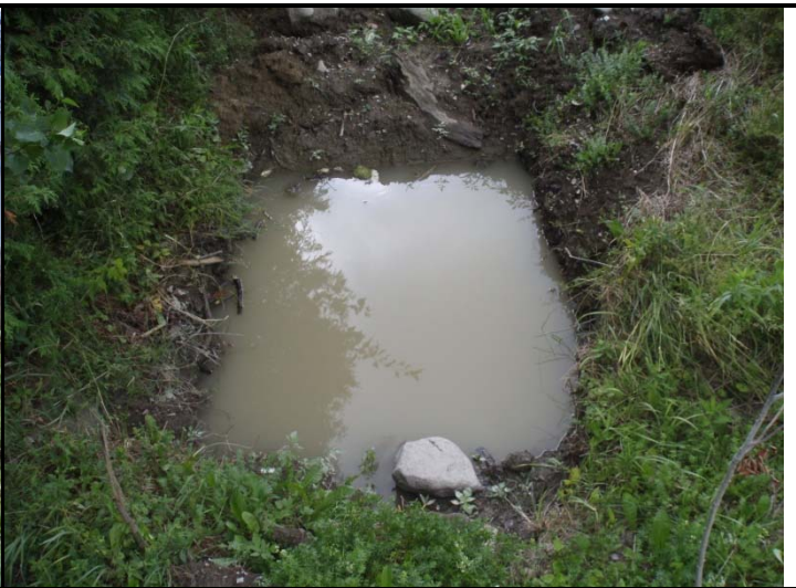
Photo 2. Close-up of submerged outfall
