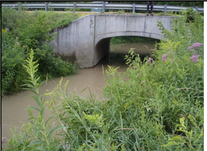
Photo 2. Upstream of bridge
