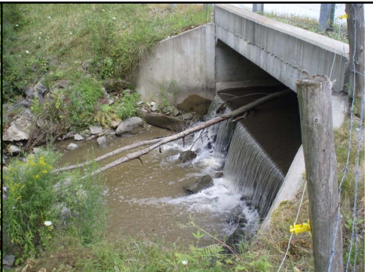
Photo 2. Downstream of bridge
