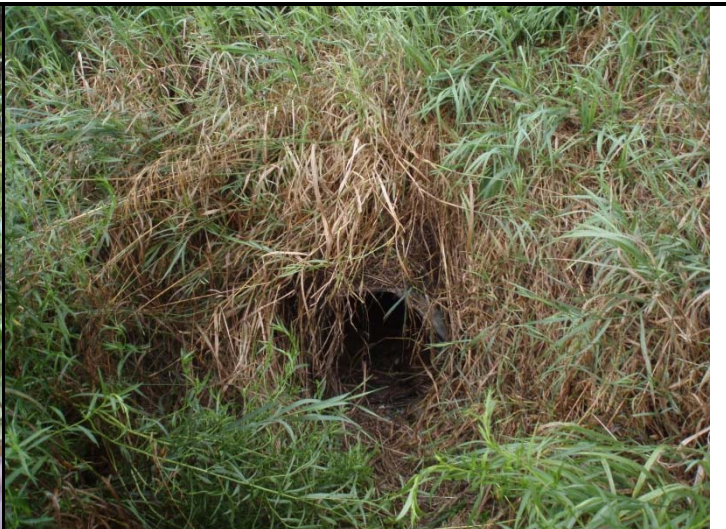
Photo 2. Upstream culvert in dense veg. of road ditch
