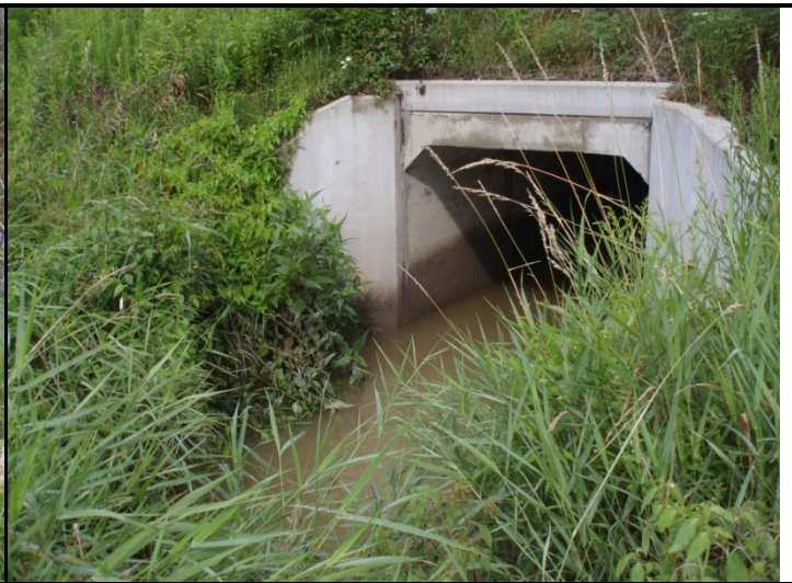
Photo 2. Upstream of bridge
