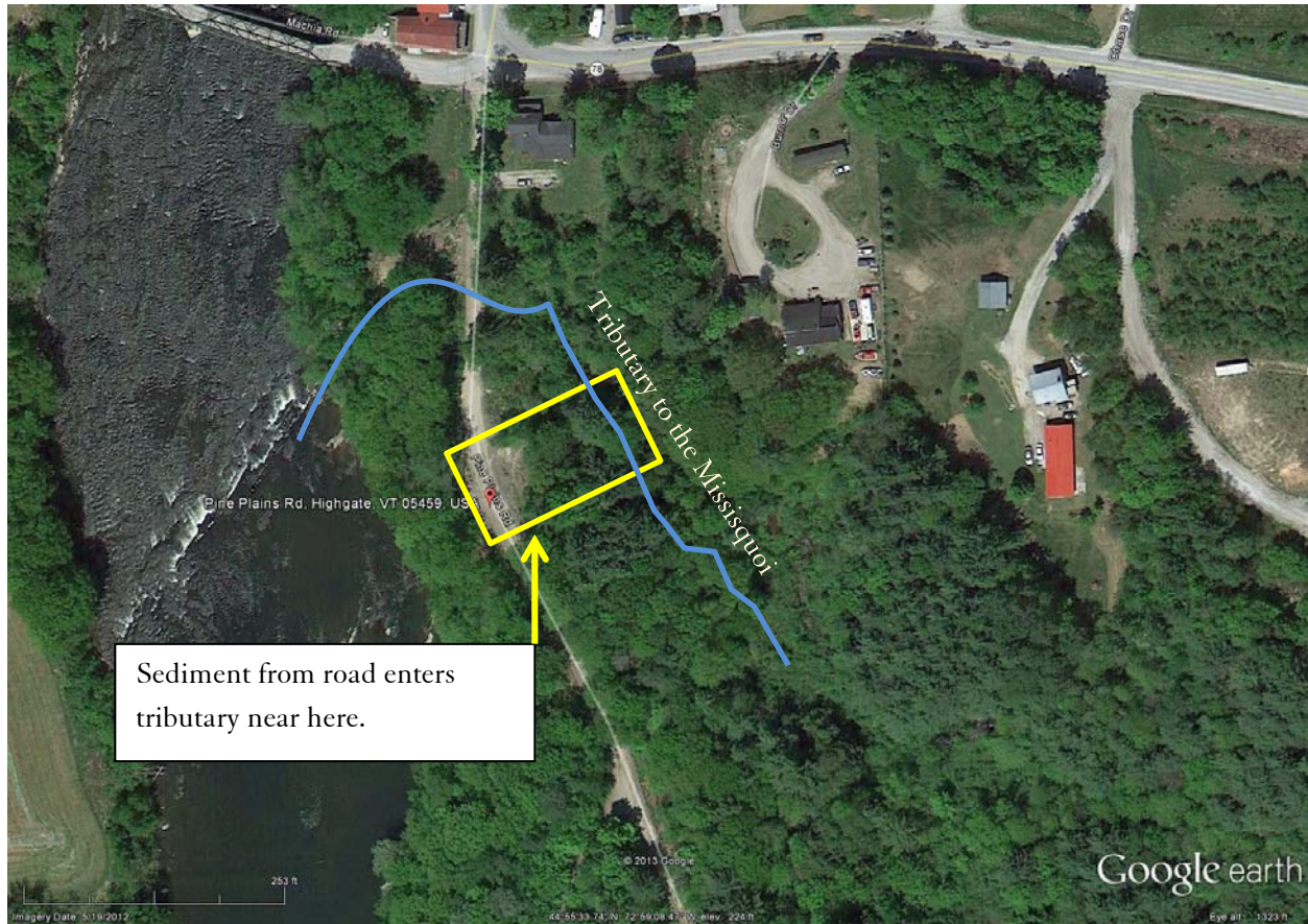
Figure 17. Pine Plains Rd. (south of VT-78) is poorly maintained. Eroding sediment from the road is impacting a tributary near the confluence with the Missisquoi River.
