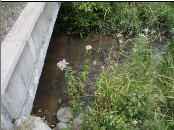
Photo 1. Upstream of bridge
