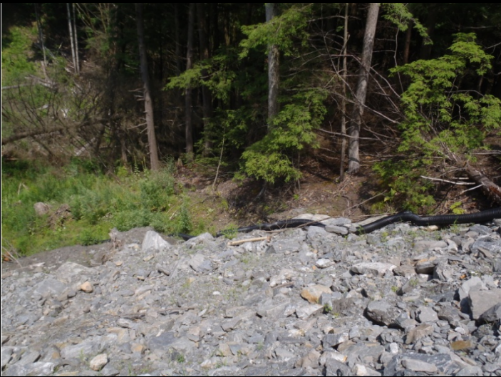
Photo 5. Pipe that now drains parking lot area
